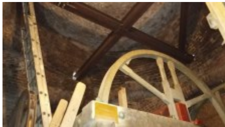
Temporary lifting beams are overhead with a bell wheel in front
