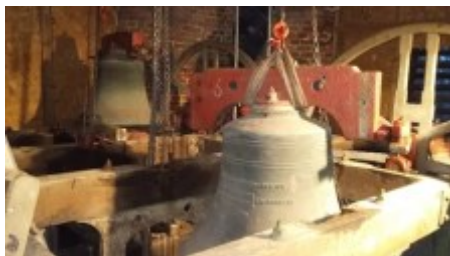
The 6 bell is lifted out of the way so part of the frame could be moved clear of the hatch
